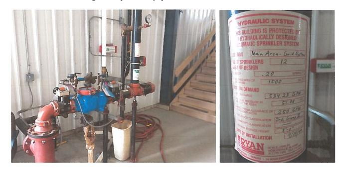
The system is designed for Ordinary Hazard Group II, which satisfies the contents and operations inside this facility. System is designed to provide 0.20 gpm over area of 1,500 square feet with a system demand of 534.23 gpm with 51.06 psi at the base of the riser. Sprinkler system is maintained, serviced and tested by Ryan Fire Protection, Inc.
