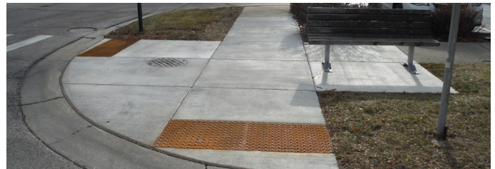
Tactile tile strips at a crosswalk in Skokie, IL
